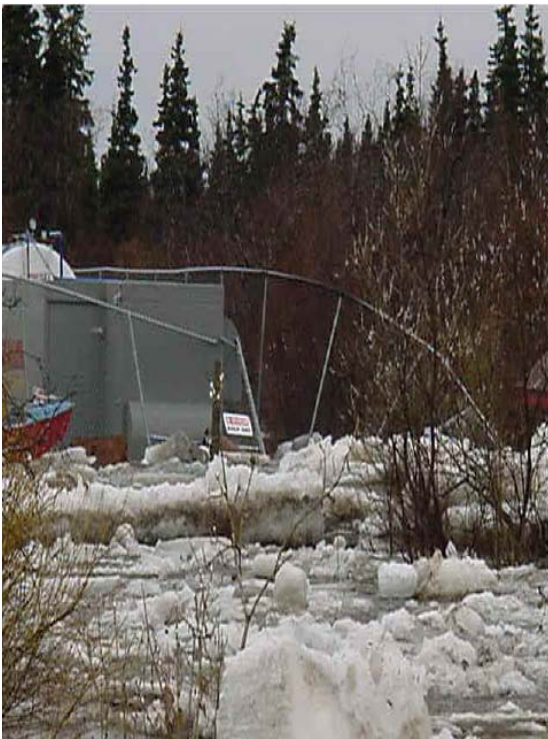
Photo 3: Ice jam pushed up around power plant, May 2002.
