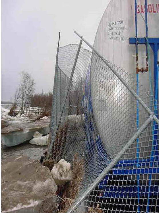
Photo 2: Fence around the power plant and fuel tanks damaged by ice jam in May 2002.
