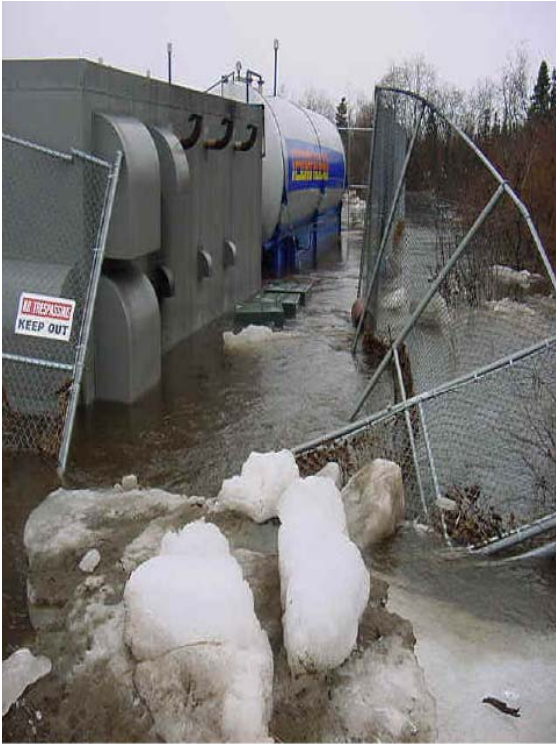
Photo 1: Ice jam flooding around the Ekwok power plant, May 2002.
